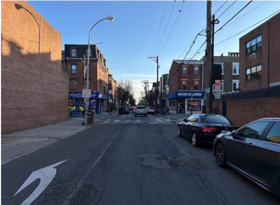
Direction / Road: Sb. S 8th Street Approach / Departure: Approach Distance: 50 feet
